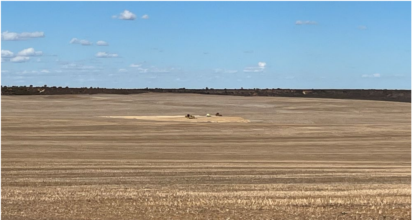
Figure 1 Booth Well Pad nearing completion
