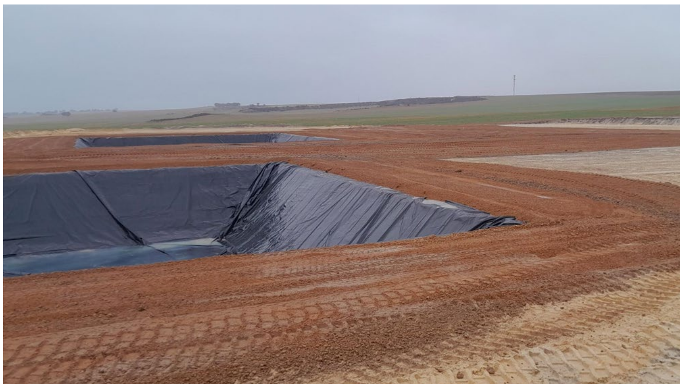
Figure 3 Booth Well Pad showing water and mud pits with waterproof lining
